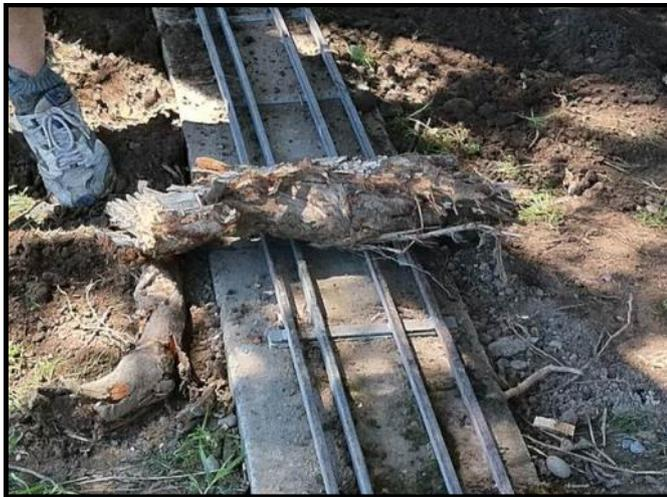
The concrete slab dropped back onto the registers and the holes were back-filled. So after four hours 'hard labour' and with a bit of skin missing from our knuckles, and a blister or two, the rails again had a true alignment giving a degree of satisfaction to those involved.
