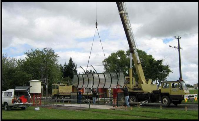
truck and unload on site placing the top onto the base which was then secured to the platform using trubolts.
