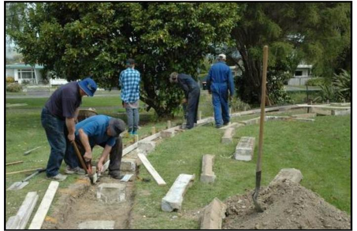
cold galvanizing paint, drilled for fastening and new conveyor belt packers glued to each sleeper. The existing concrete base was dealt to with an electric Kango Hammer. The boxing
