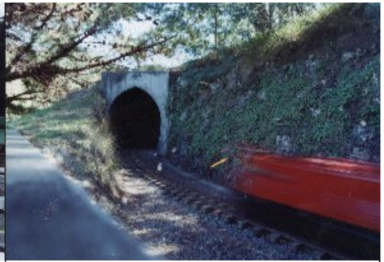
Colin's "EC" speeds between Tunnel 2 & 3
