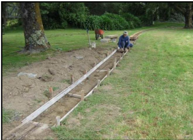
On the 12 Nov 2010 the concreting was done, A cubic metre of concrete delivered to the site in one of Higgins trucks was quickly placed, screeded and troweled off and in a weeks time the boxing will be removed and the rails will be bolted back down.
