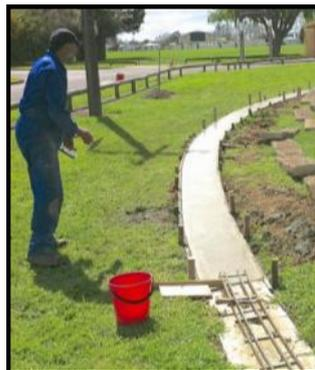
Monday 16th September saw the concrete truck on site and in a very short time the concrete was placed, screeded and edged by much the same team. Friday 27th the track was re-laid after the boxing was removed and the ground along the
