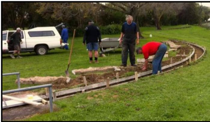
The next day the team size increased with Brian and Warick Leslie, Richard Lockett, Graham Toms and Chris Morton joining in. The old concrete bed was cut with a concrete saw, heaved aside and boxing pegged in place.
